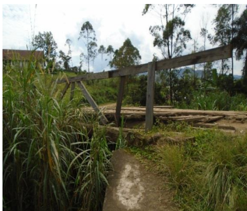
Pont WERE à Nyabiondo
